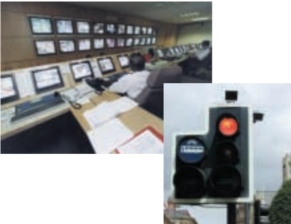
UTC Systems are being improved throughout the county.
